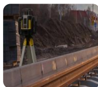
Rail 铁轨铺设
